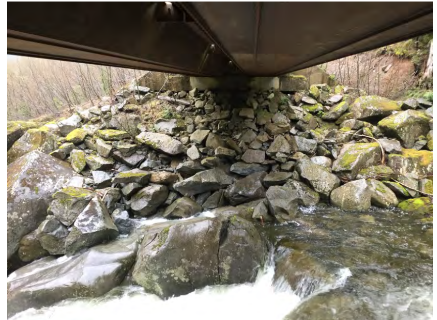
Right Bank Abutment when facing downstream
