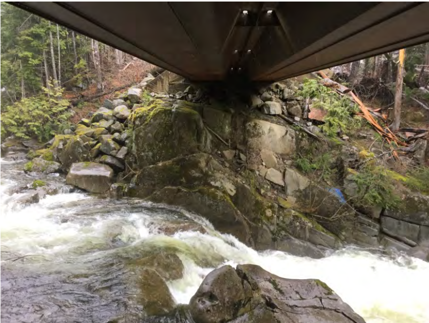
Left Bank Abutment when facing downstream
